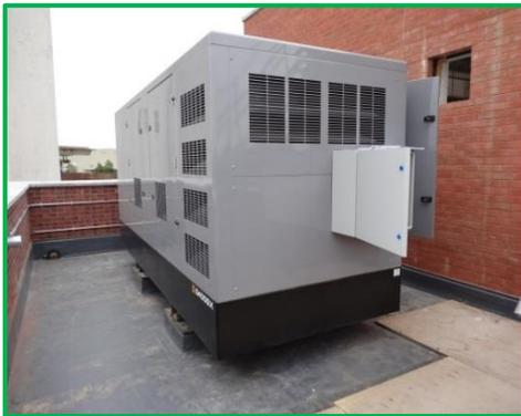
The standby generator was recently delivered and placed on the first floor roof. The generator is a backup source contingency against a loss of mains power when closing the barrier; ensuring that it can be operated as normal should there be a power cut. As a further failsafe there will also be diesel powered emergency power packs to drive the barrier's hydraulic system in order provide a further level of contingency should both the mains power and the generator fail.
